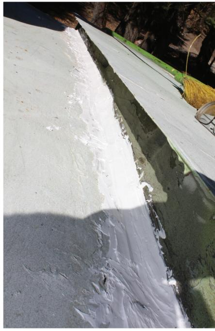
This leak allowed water to seep into the sub-roof of the building and eventually drip down directly upon the 6 meter repeater. This failed seal was stripped and redone in order to provide weather proofing for the rains that fell starting Sunday night (photo in center). The emergency water ducting previously erected in December was allowed to remain in place as a back-up (pictured below).
